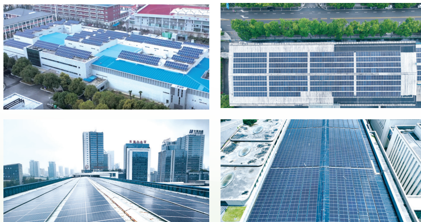
Photovoltaic system installation
