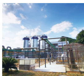
Sewage treatment system of Guilin Pharma
