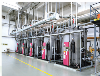
Boiler renovation of Avanc Pharma
